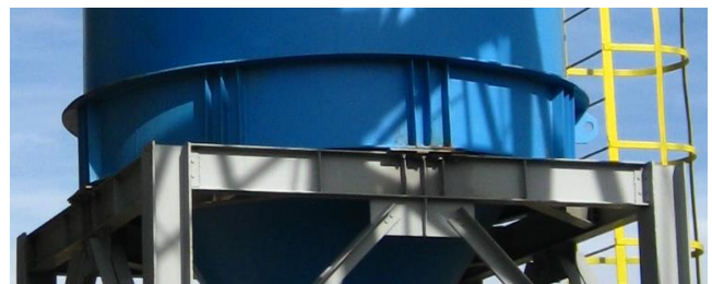
Fig. 1. Stiffeners in discrete supports of shell.
